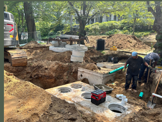
IA System Install at Locust Valley Library.
